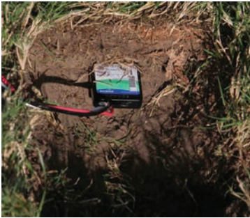
Soil Moisture Sensor Installed
